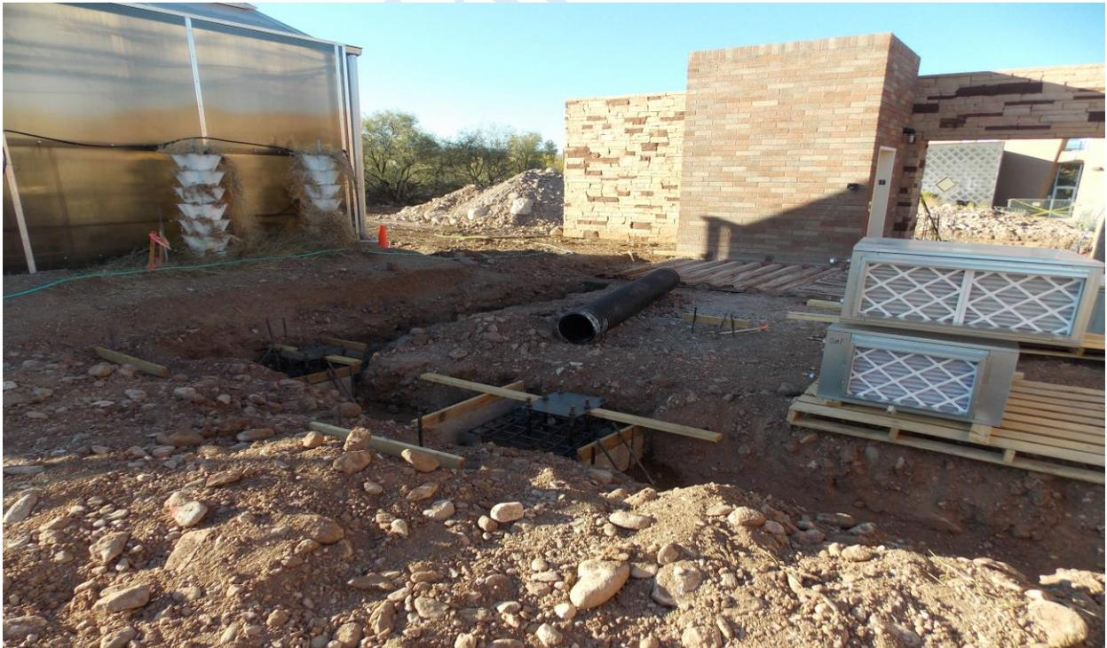
Anchor Plate and Piers for new Columns for Building Main Entrance
