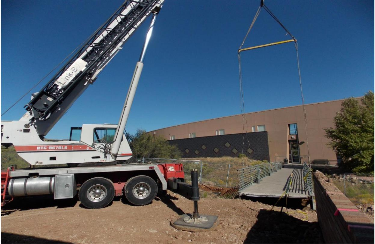
Lifting of Bridge between Buildings L and M for Structural Reinforcement
