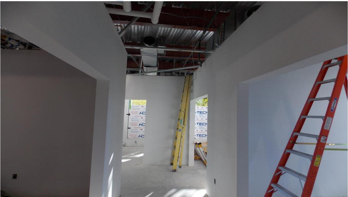
Installing Ductwork and Preparation for Ceiling Grid
