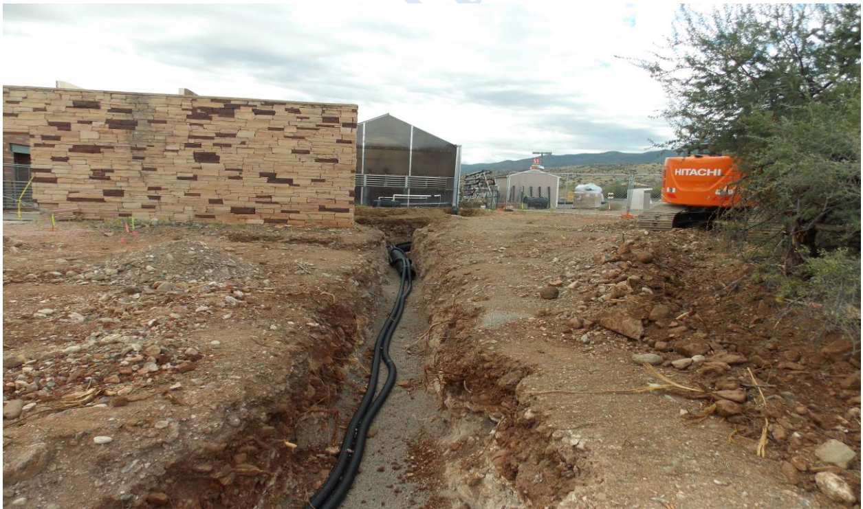
Roof Drainage
