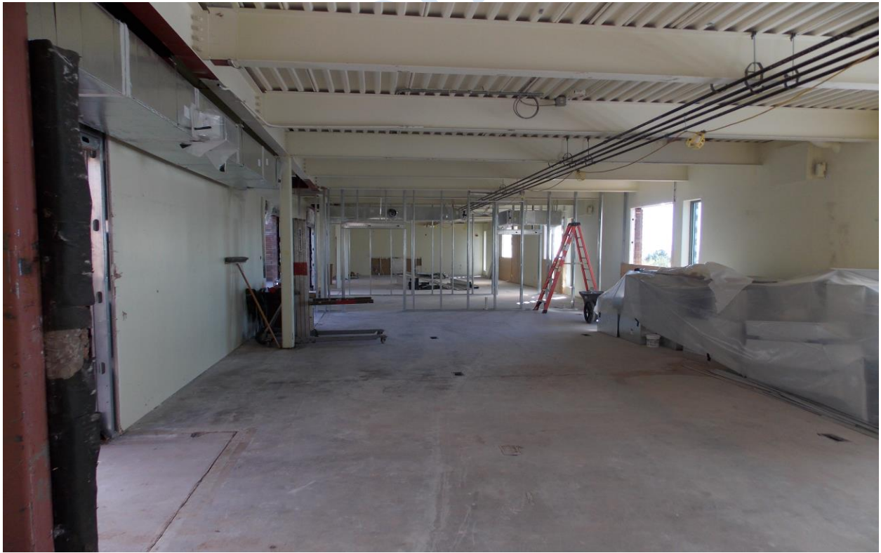
Water Recirculation Piping for Heating and Cooling
