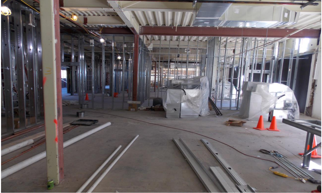
Electrical Rough-in and Mechanical Installation for Science Labs
