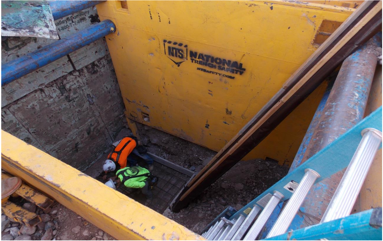
Excavation for Foundation Reinforcement
