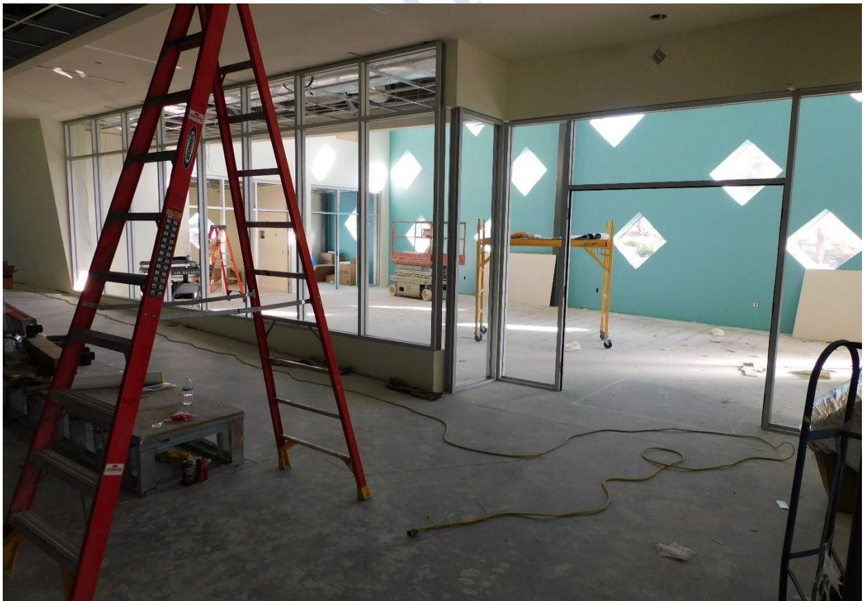
View into the Tutoring space
