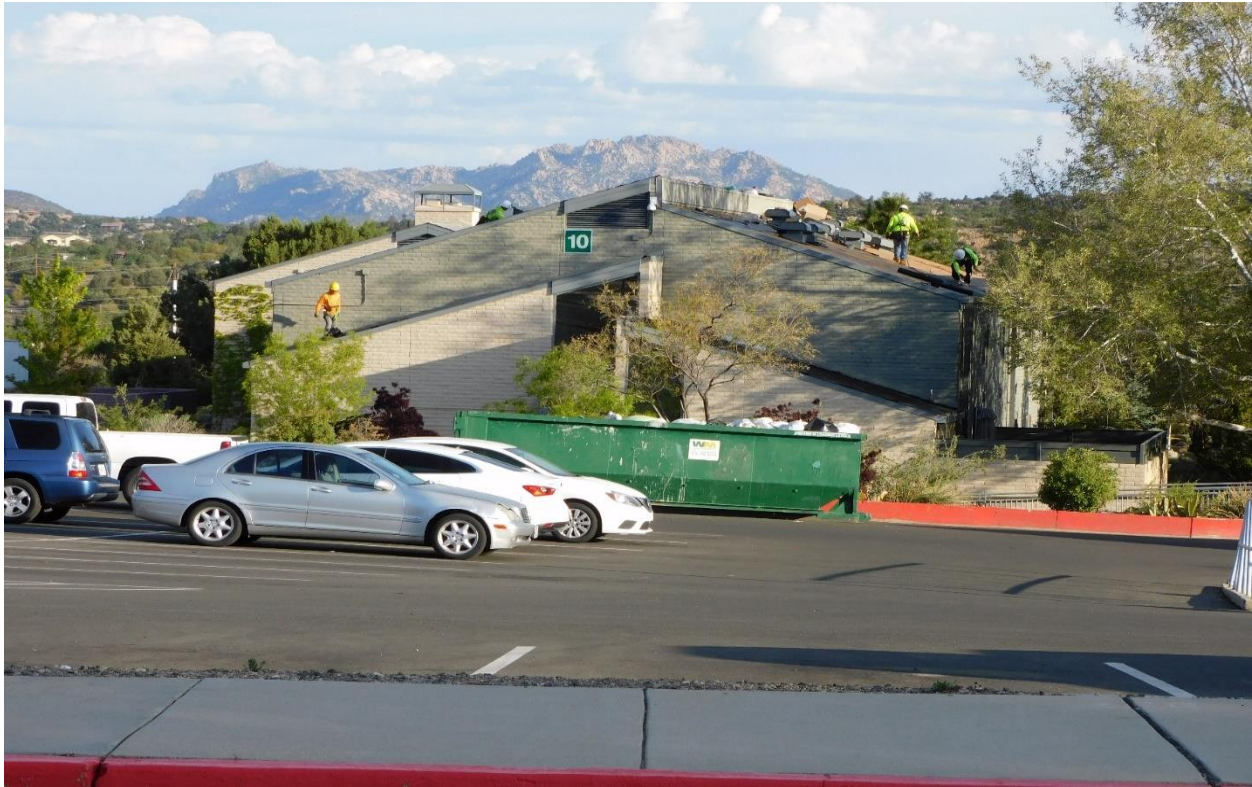
Roof replacement at Marapai Hall
