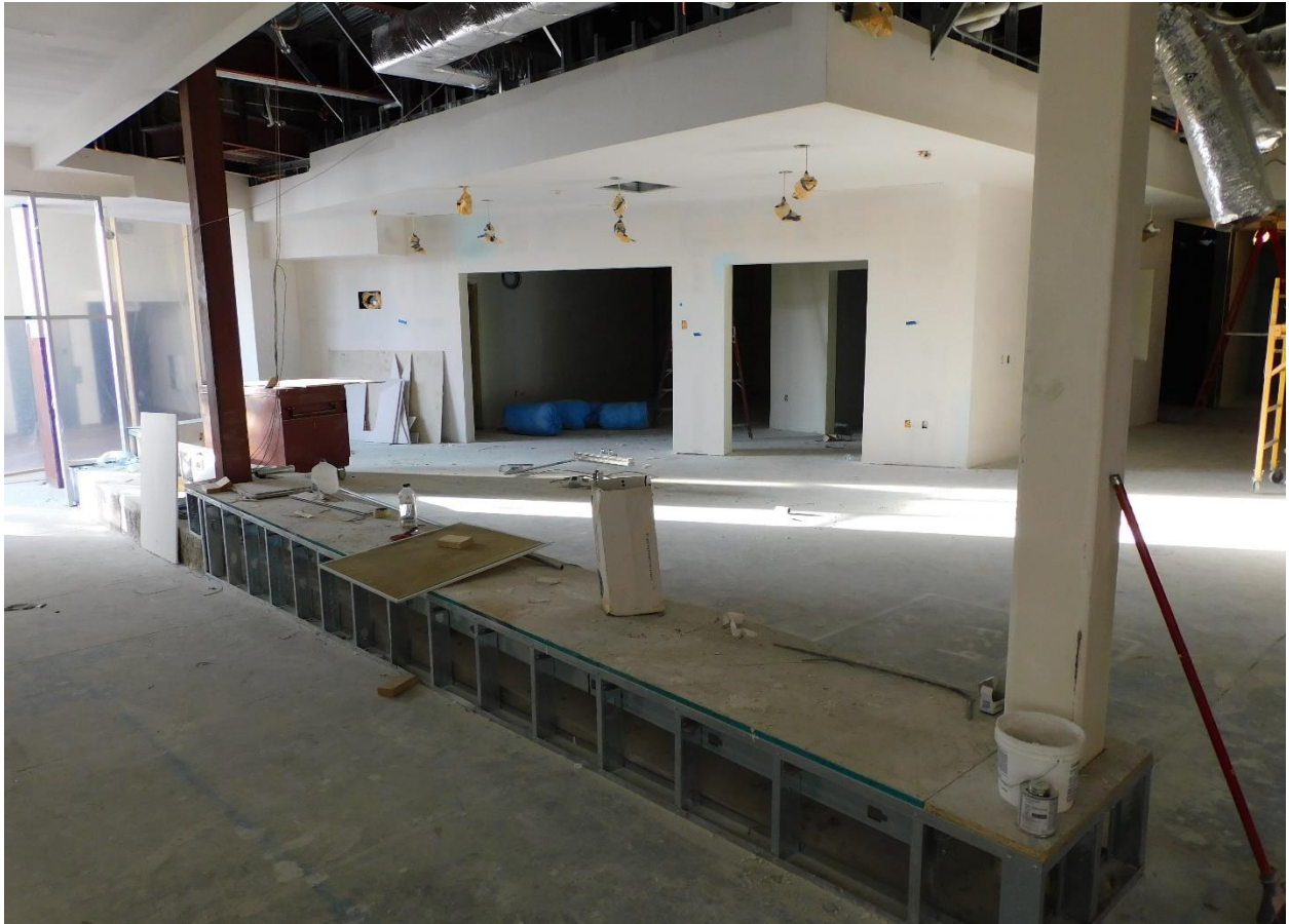
Information desk and front offices
