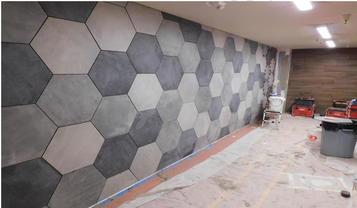
North restroom renovations at CTEC
