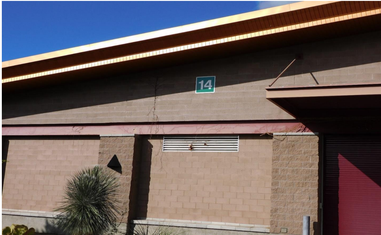
New building identification signs
