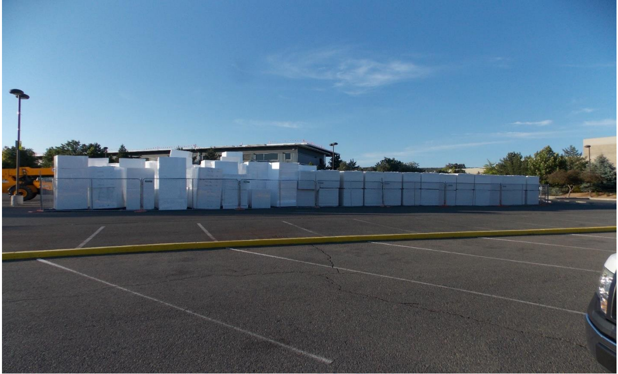
Roof Insulation for Building 19
