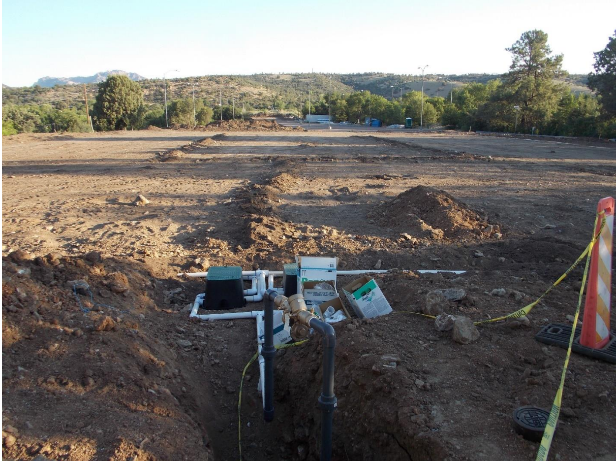
Backflow preventer and assorted irrigation valving
