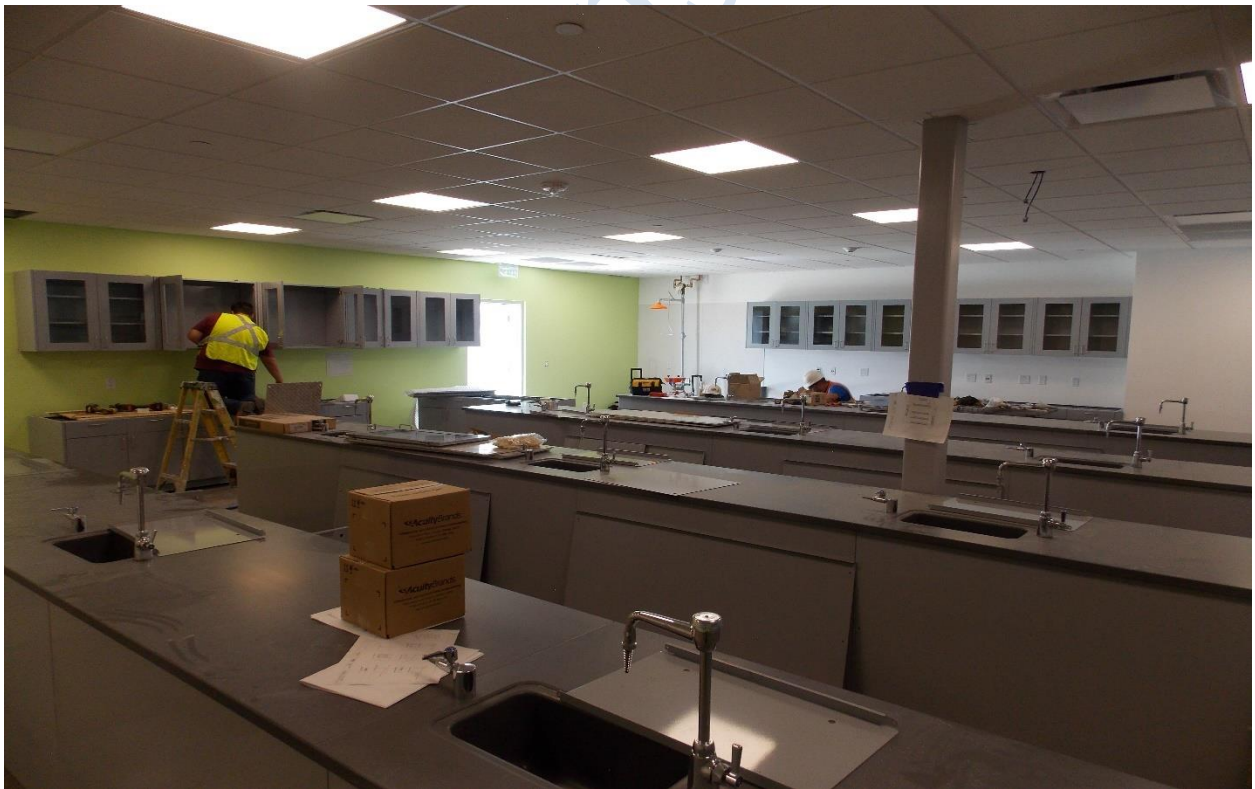
Millwork installation in the science lab
