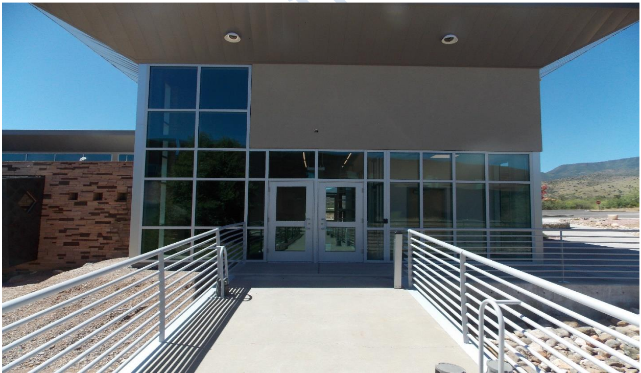
South entrance from Building M
