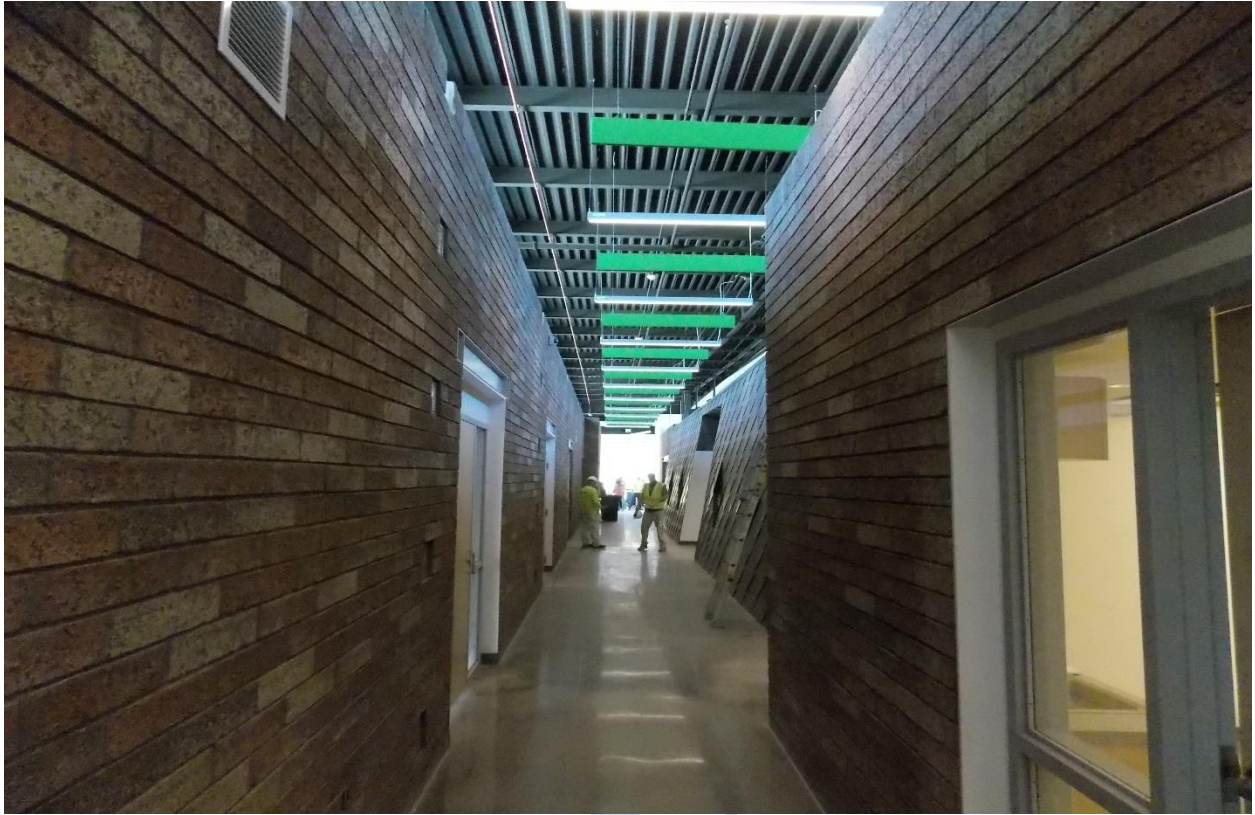
New lighting in second-floor hallway
