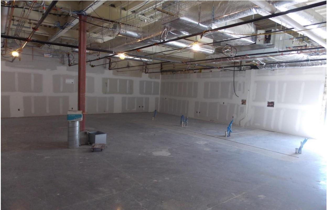
Drywall mud and tape and diamond plate utility chase installed in Biology Lab
