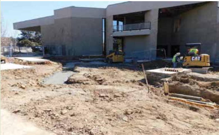
Construction started for the Technical Theater, Prescott Campus
