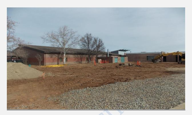
Installing New (Yellow) Gas Line for Central Plant
