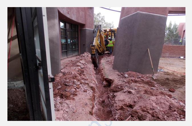
Use of 1,000 Pound Backhoe Hammer to Break Rock for Culinary Waste Grease Line
