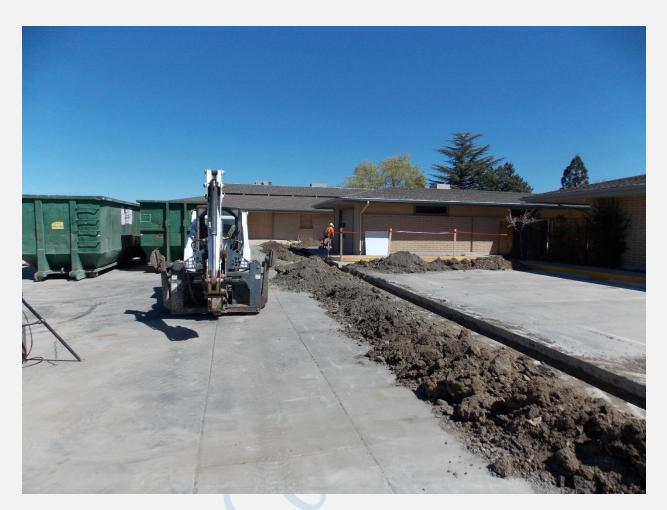
Trenching and Saw Cutting for Buildings 30 and 31 New Water Line
