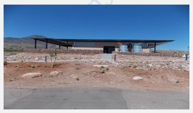
SWC East Elevation with Rain Water Capturing Storage
