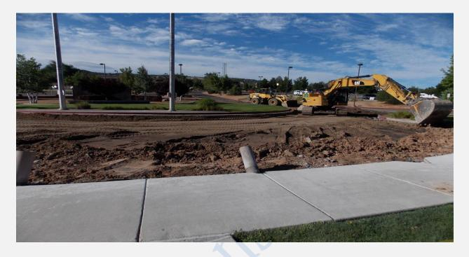
Replacing Damaged Asphalt with Concrete at Traffic Circle Prescott Campus
