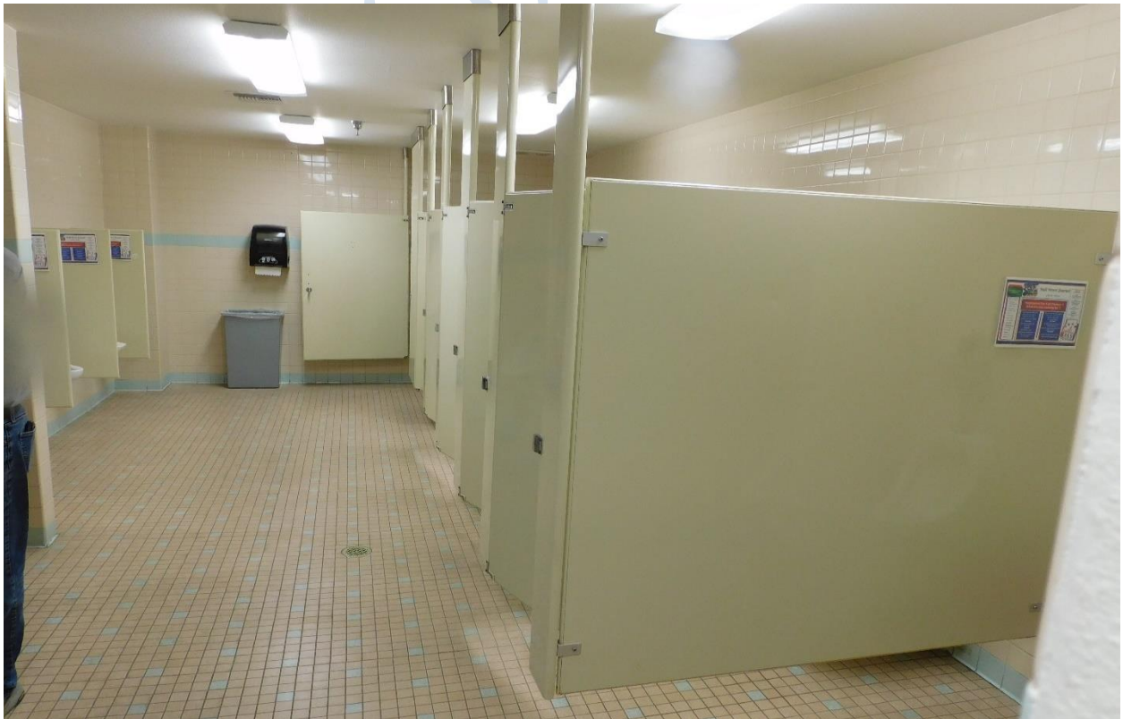
CTEC restroom before rehabilitation
