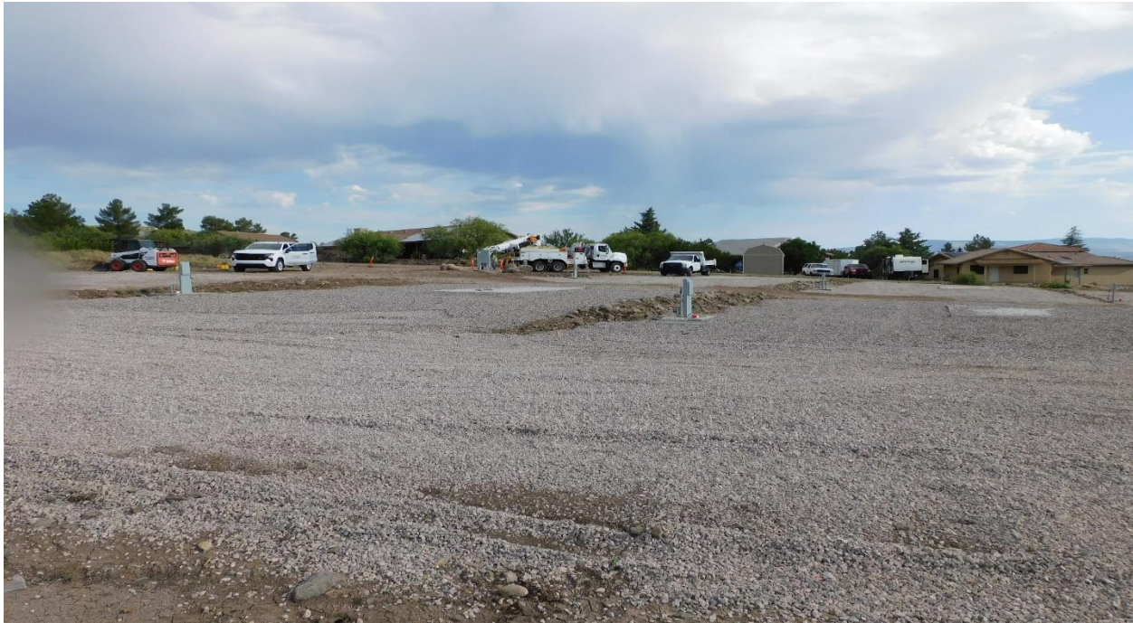
APS installing electrical service to RV pads
