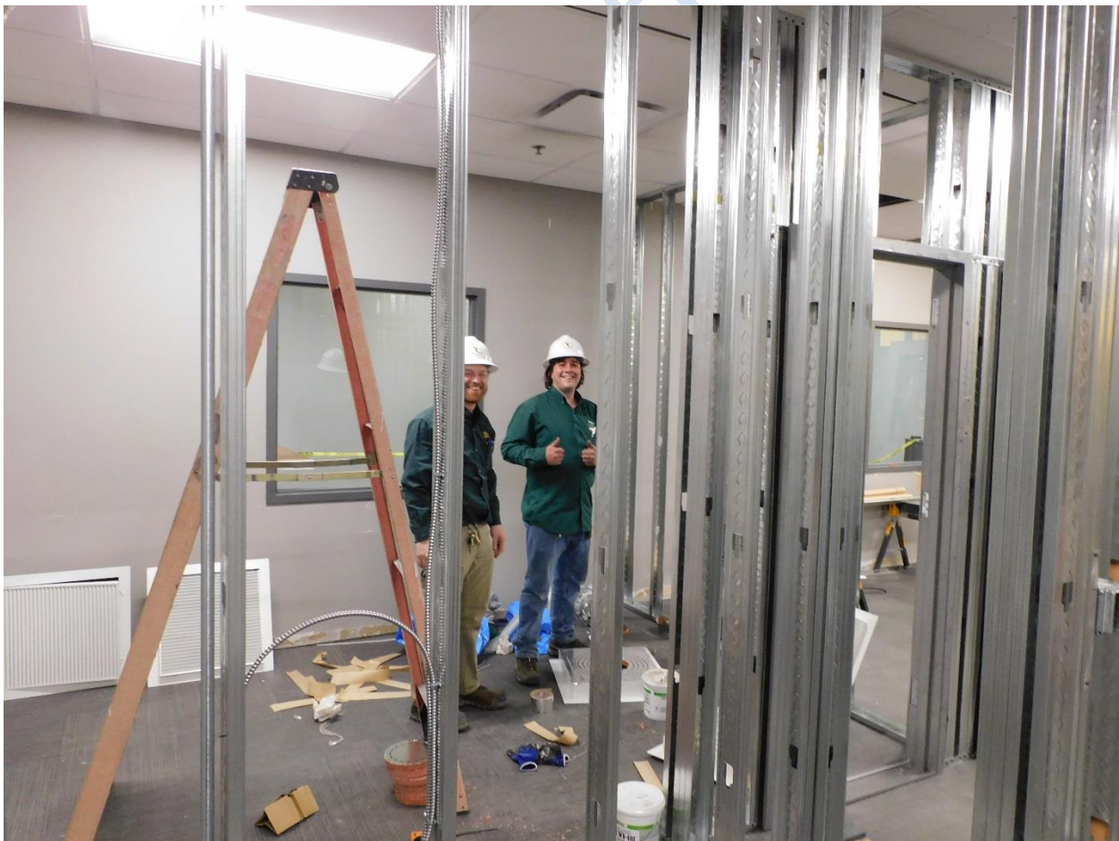
HVAC Team members Ben Blumstein and Brandon Hopper-Barraza installing registers
