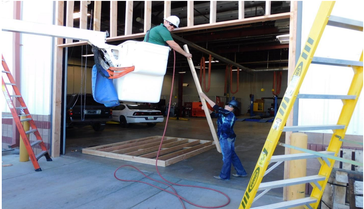
Ms. Stephanie assists Brandon Biro in framing a new door at Automotive
