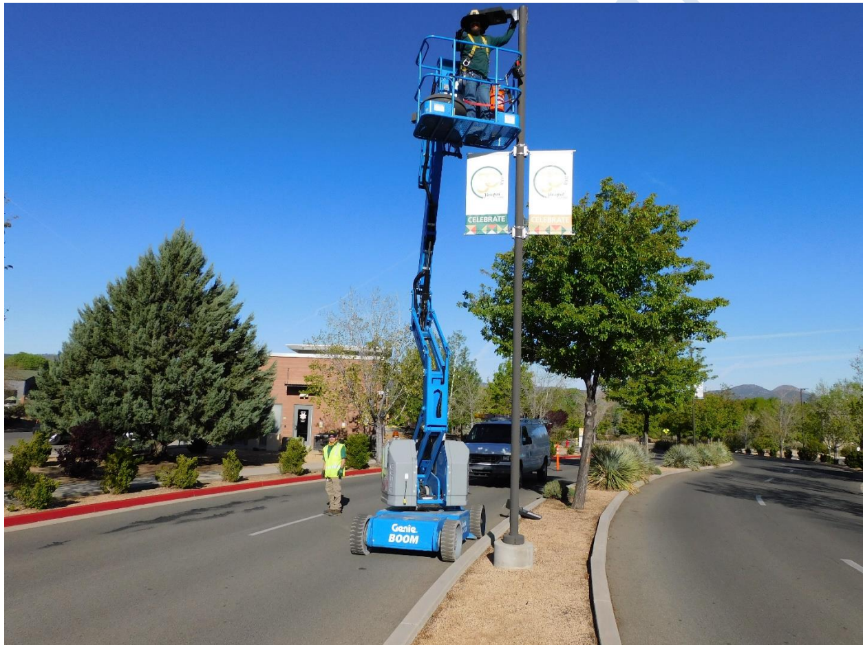
Electricians Don Stevens directing traffic and Zack Vannoy installing LED lighting
