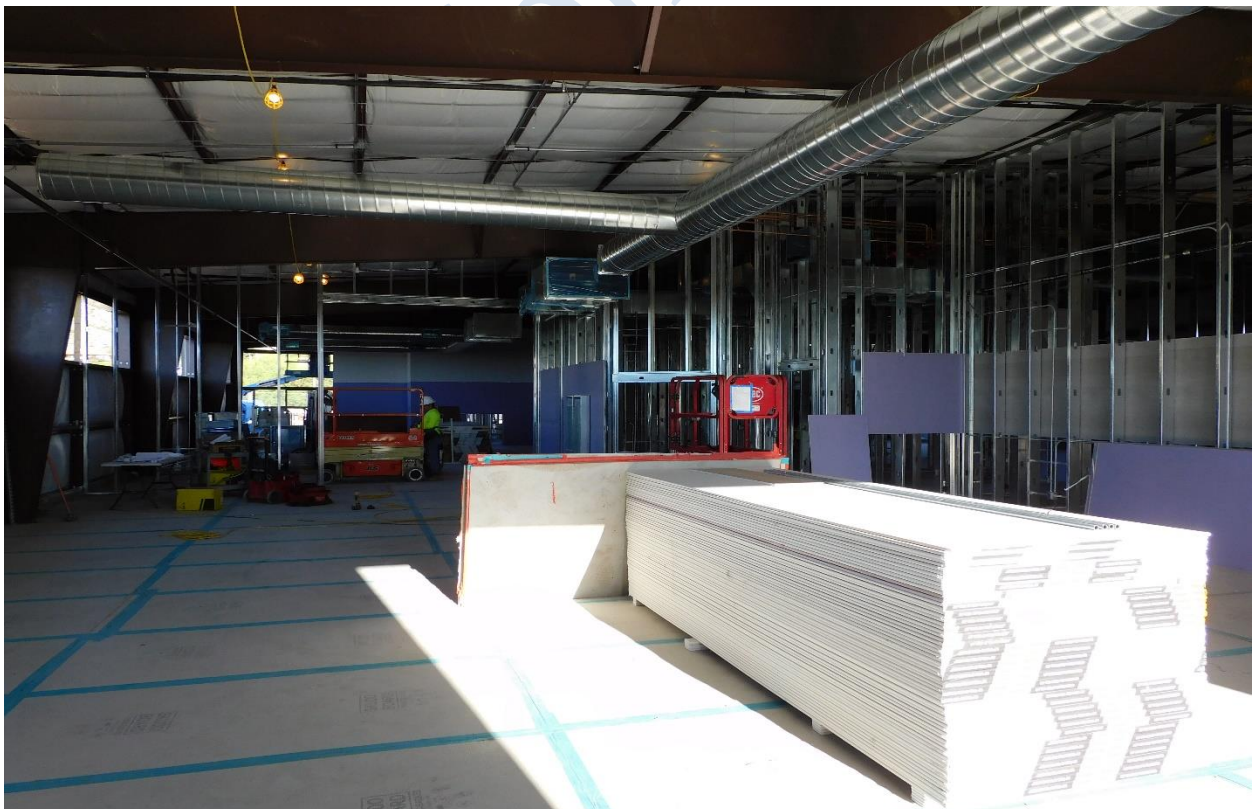
Installing wall paneling in the HVAC Lab
