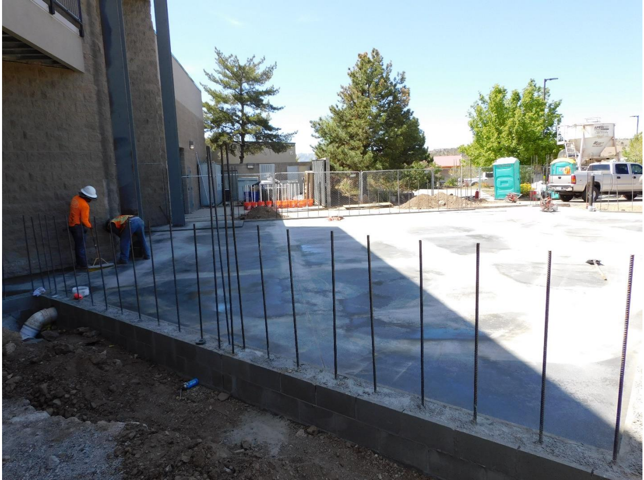
Stem wall and new slab
