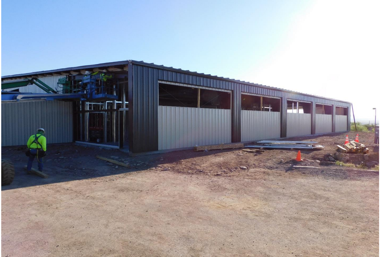
Installing metal panels on the south side of the building
