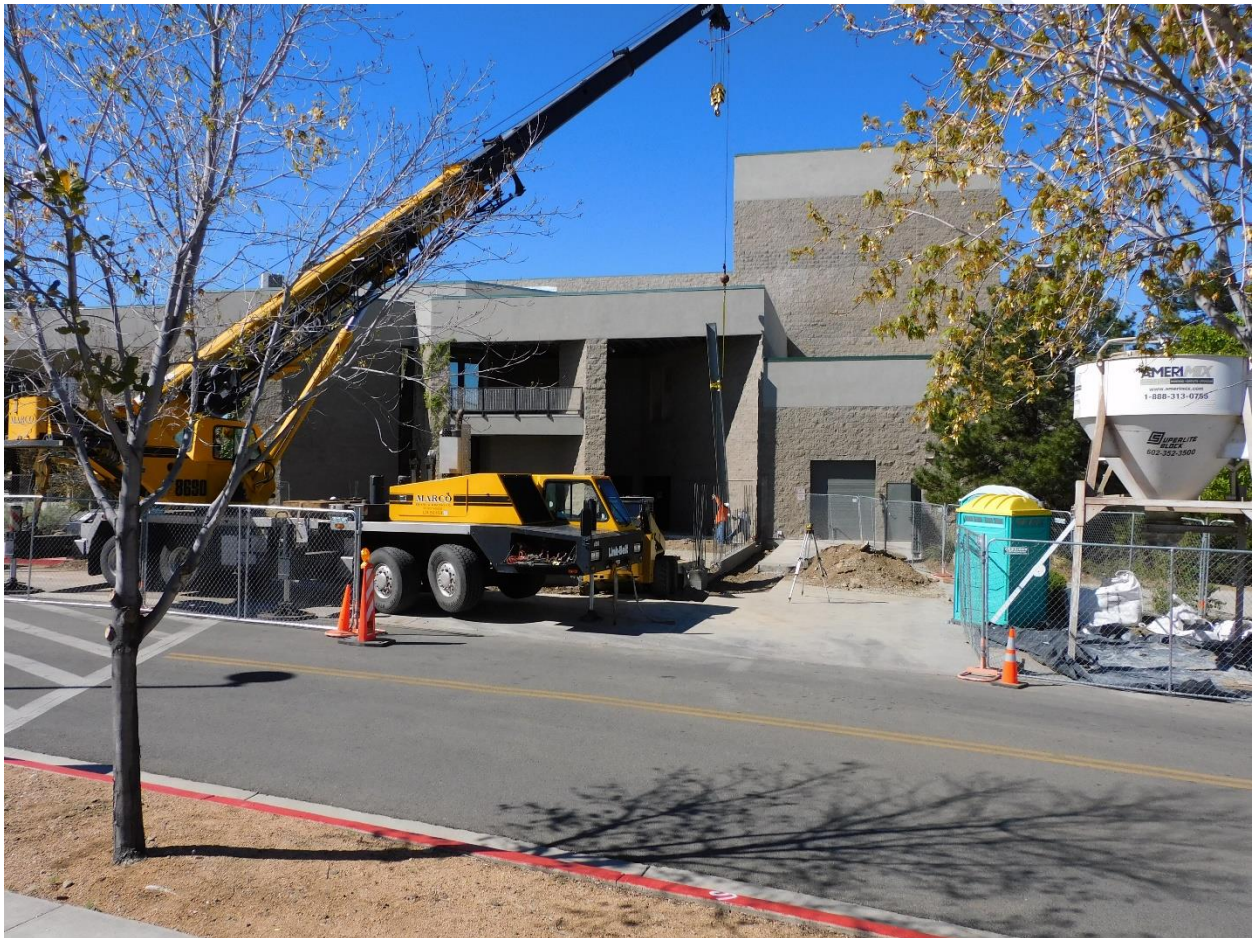
Setting columns to support mezzanine space
