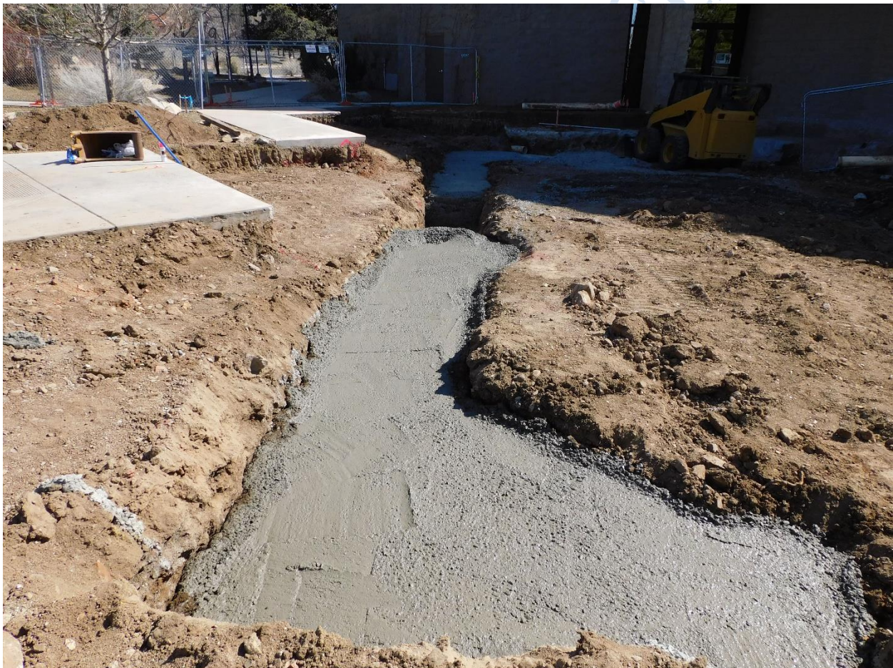
Close up of footers to support new walls for Technical Theater
