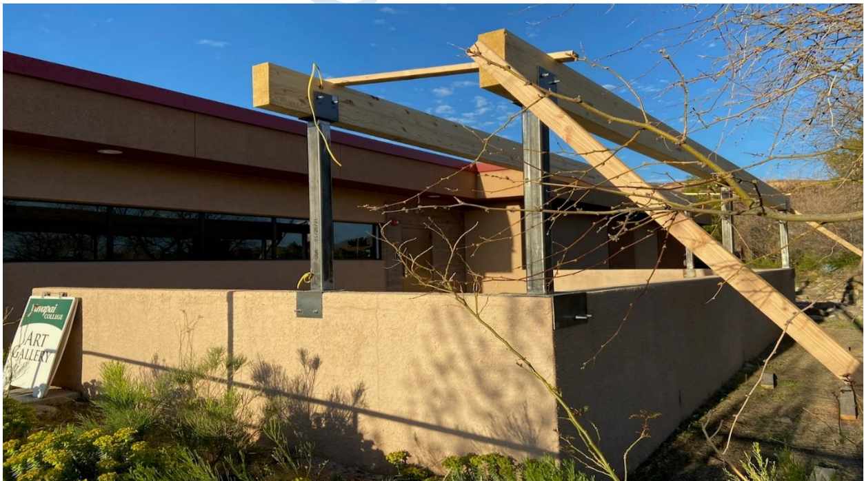
Structure columns and glue-laminated beams for the pergola
