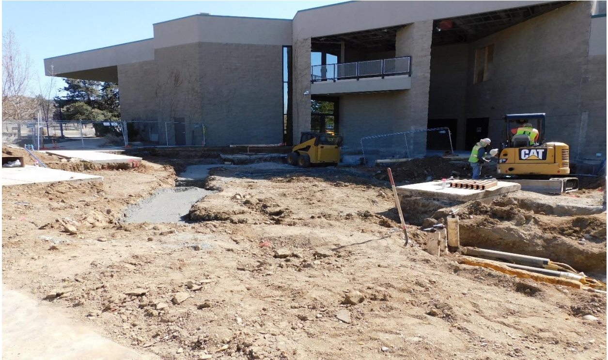
Site excavation for new footers and concrete floor
