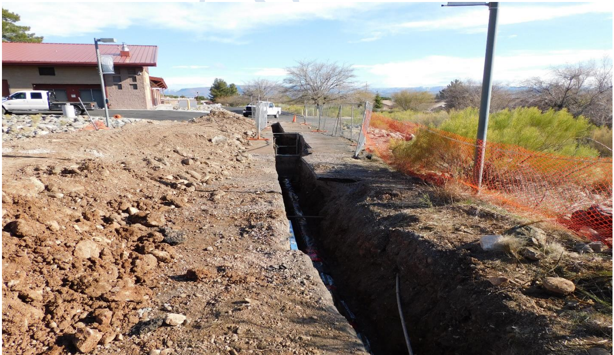
The new water line from building A
