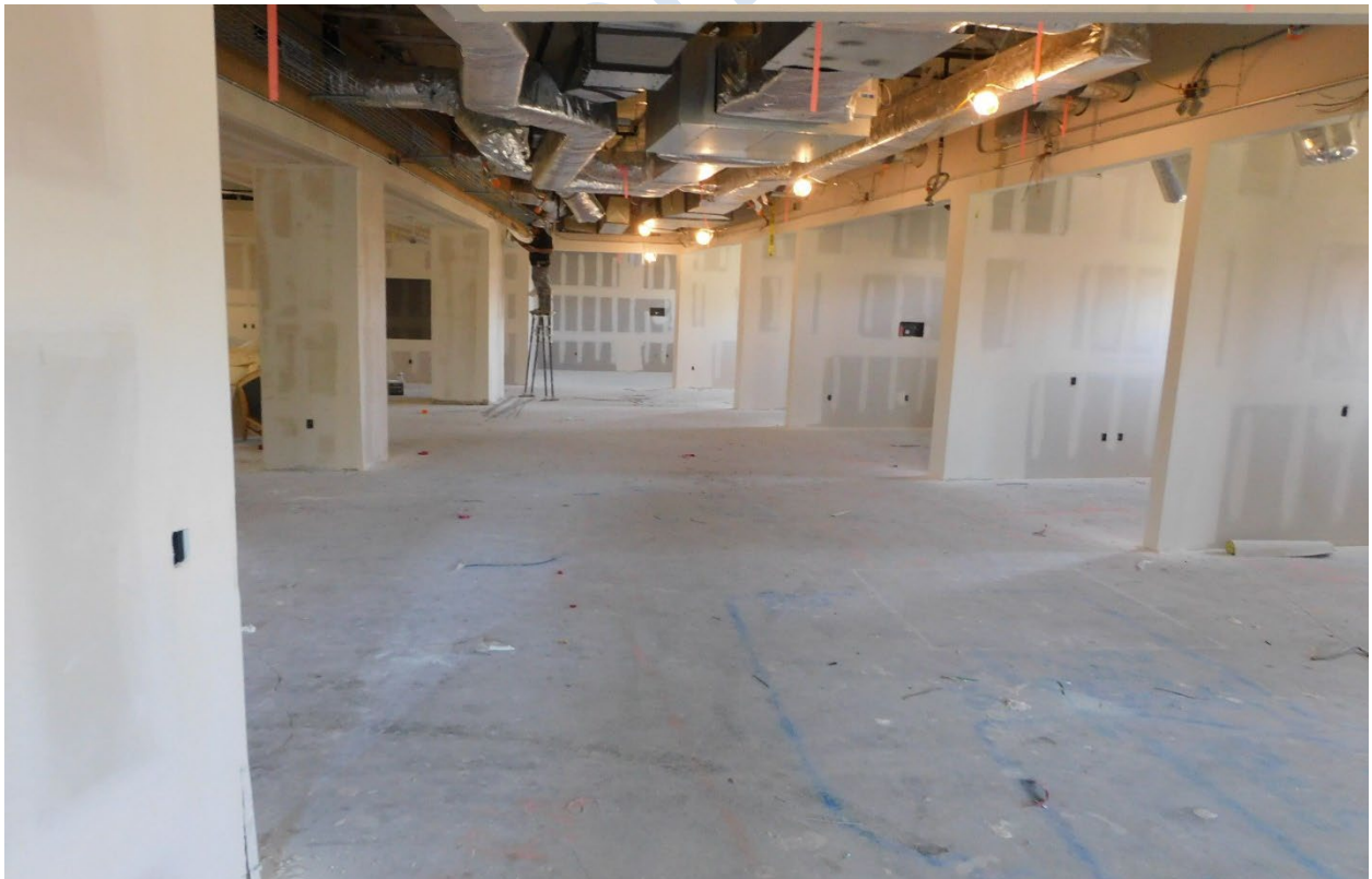
Prepping for paint and new ductwork in breakout rooms
