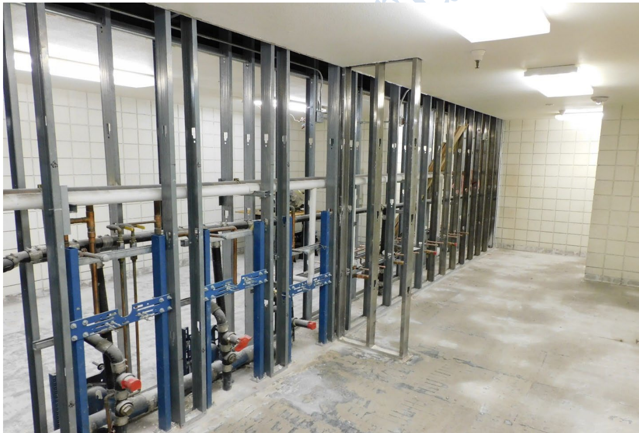
North restroom renovations at CTEC
