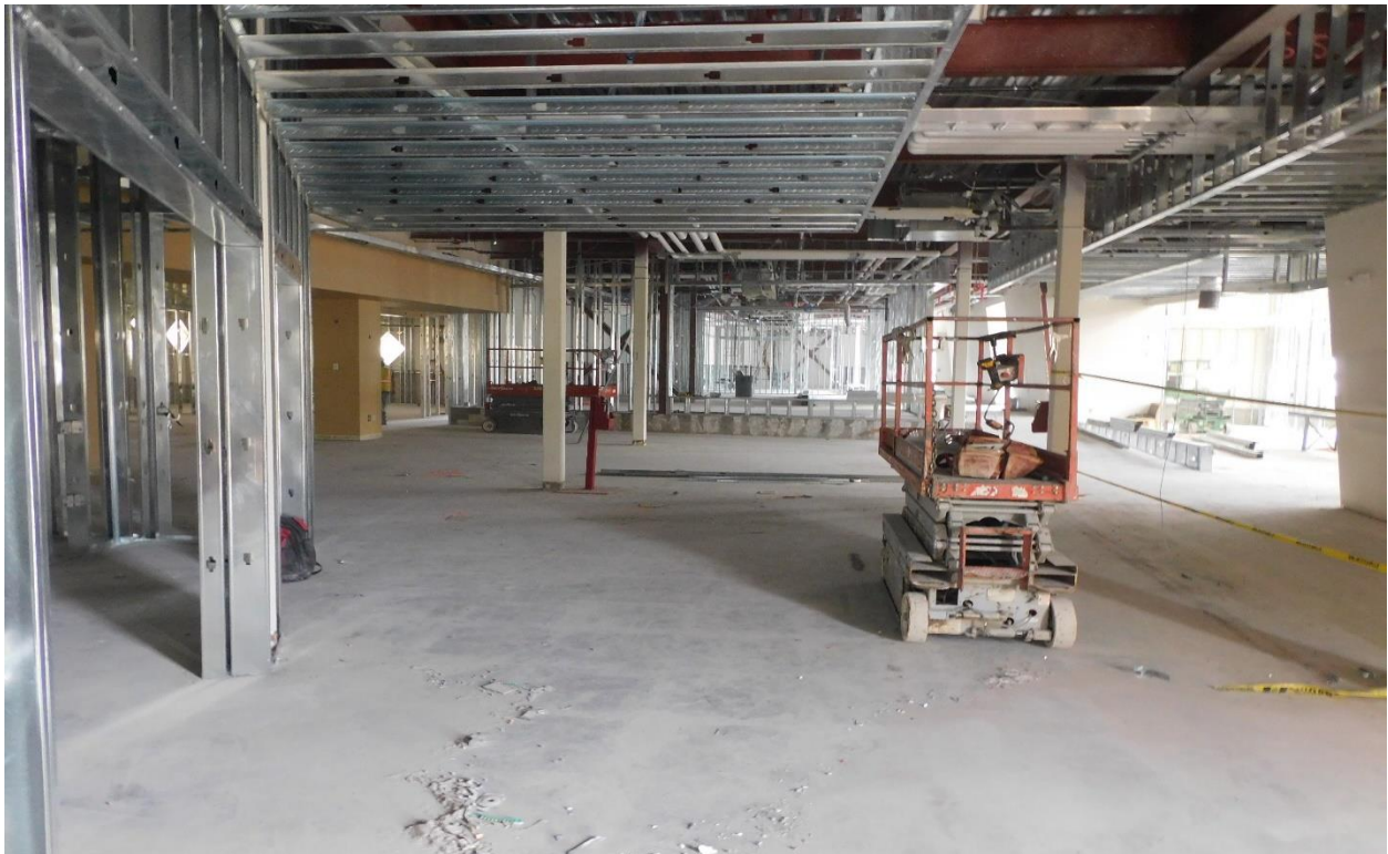
Information desk to be located to the left, tutoring and group study spaces to the right
