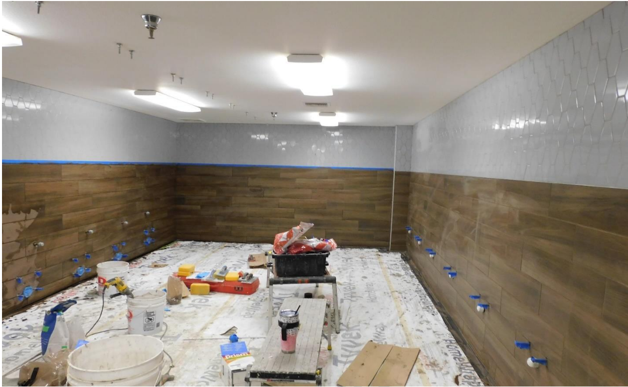
CTEC restroom rehabilitation
