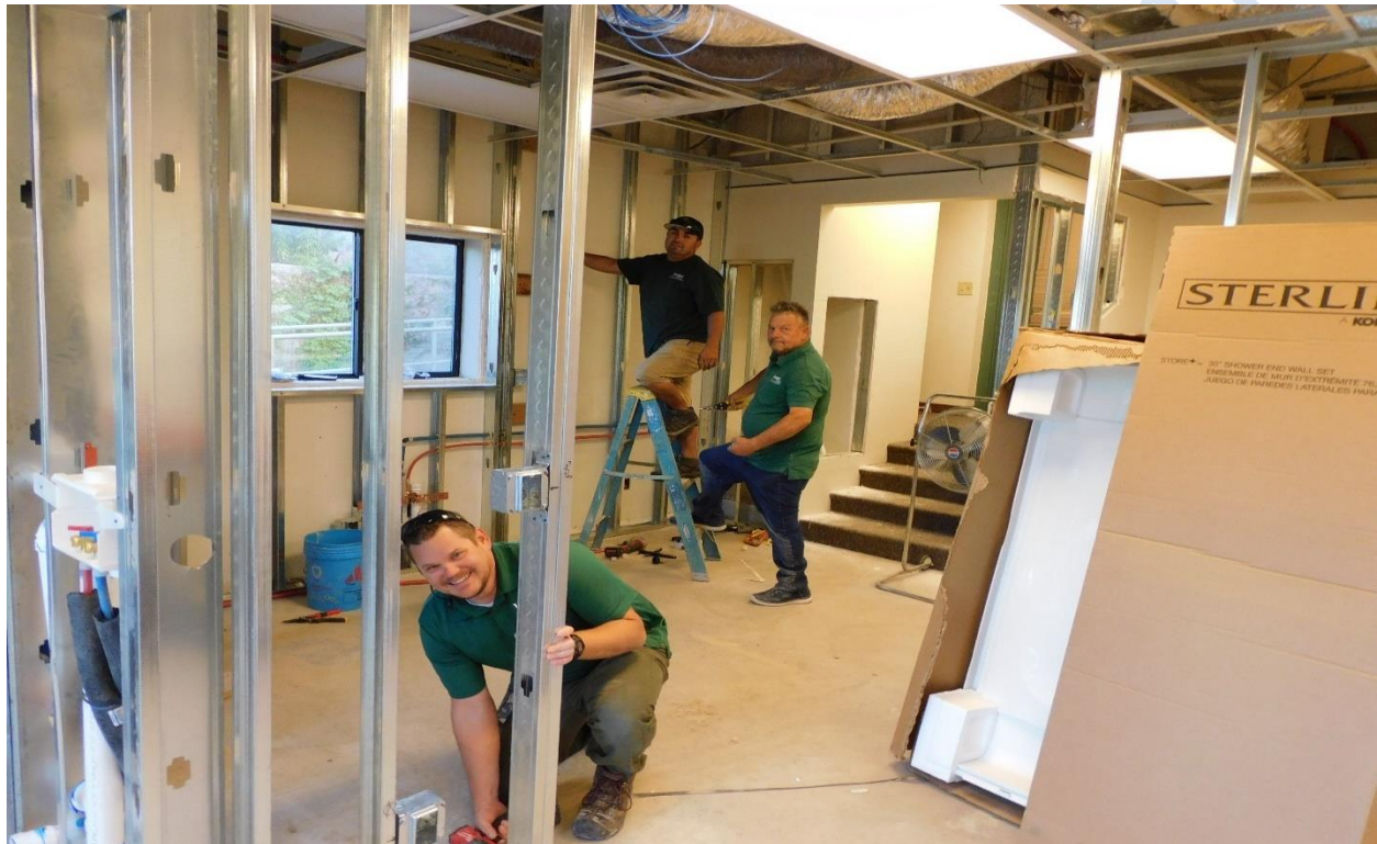
Brandon Biro, Jaime Hernandez, and Michael Murphy Building 34 apartment conversion
