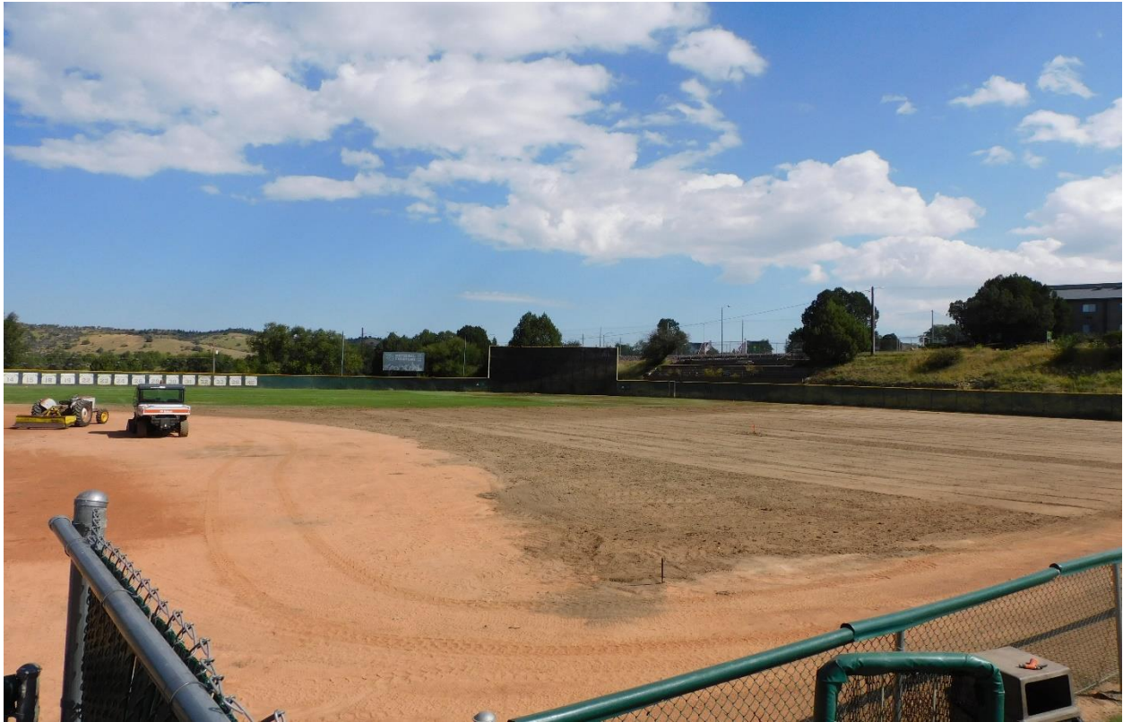
Site leveling in preparation for new sod
