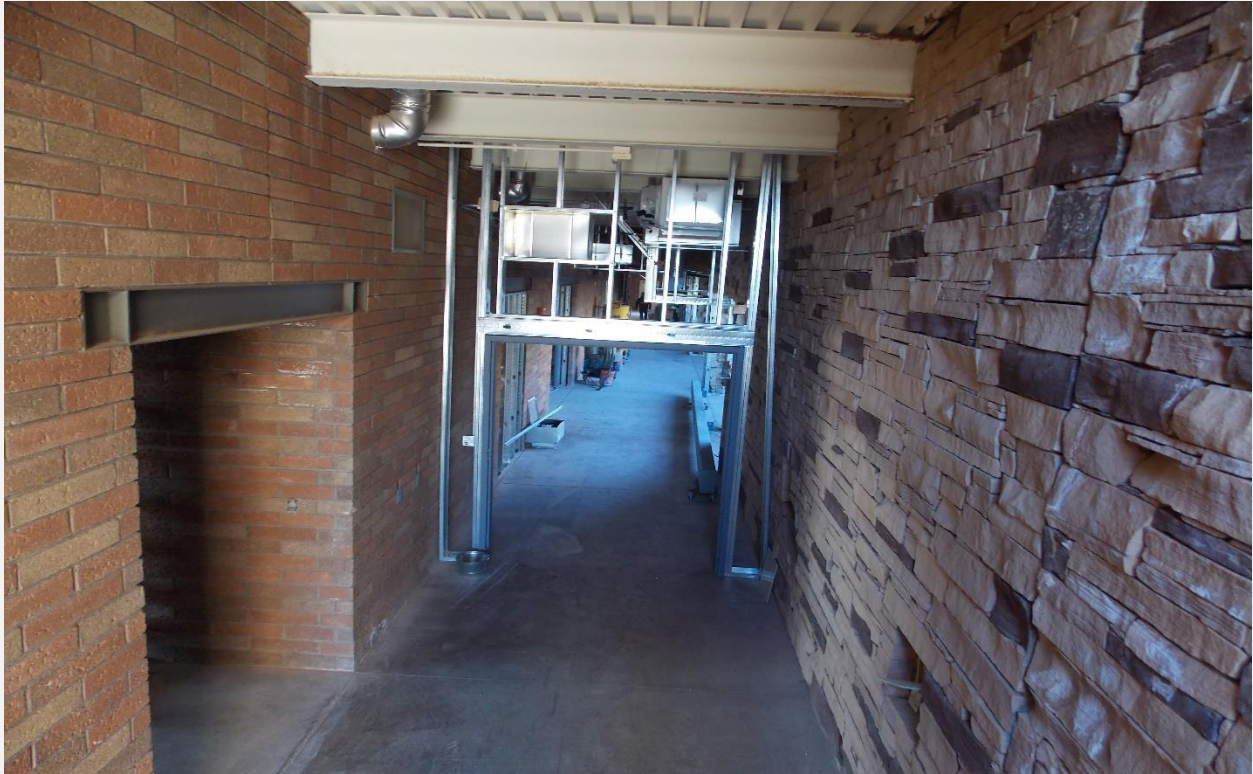
Constructing New Enclosed Hallway - First Floor
