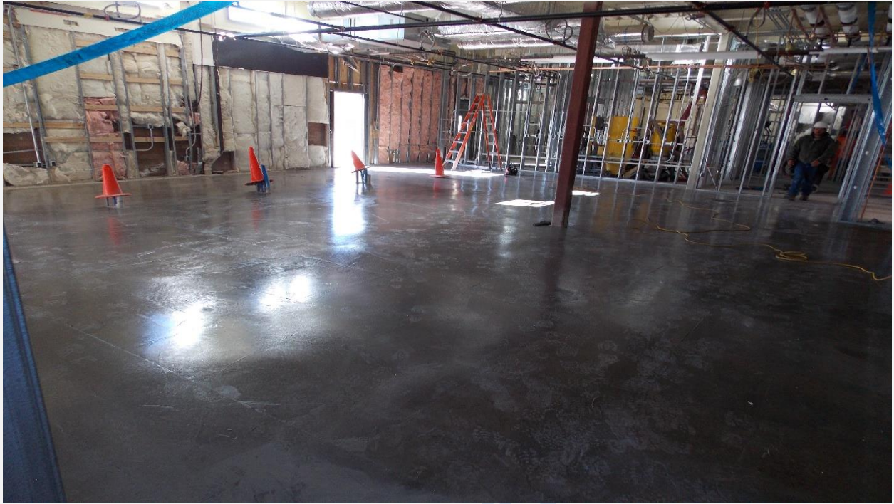
Polished Concrete at the Science Labs
