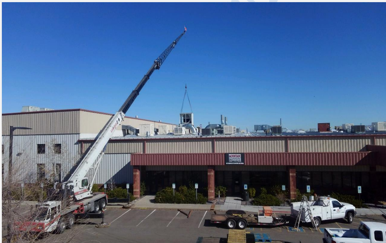
Removing Mechanical Components in Preparation for Roof Coating at CTEC
