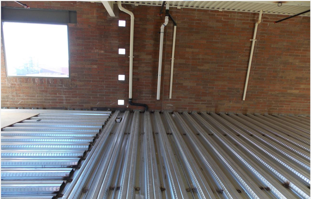
New Decking at Simulator Labs Above Advanced Manufacturing
