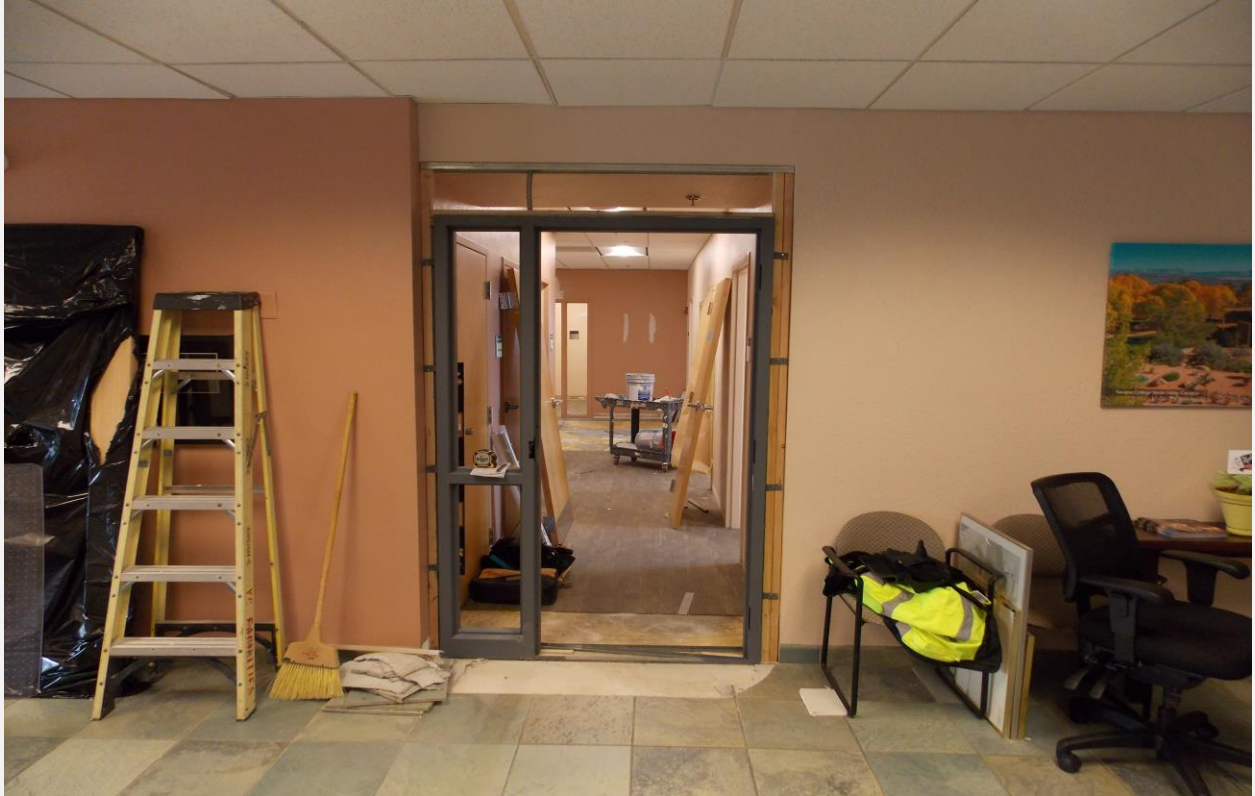
Lobby and West end of Building 32
