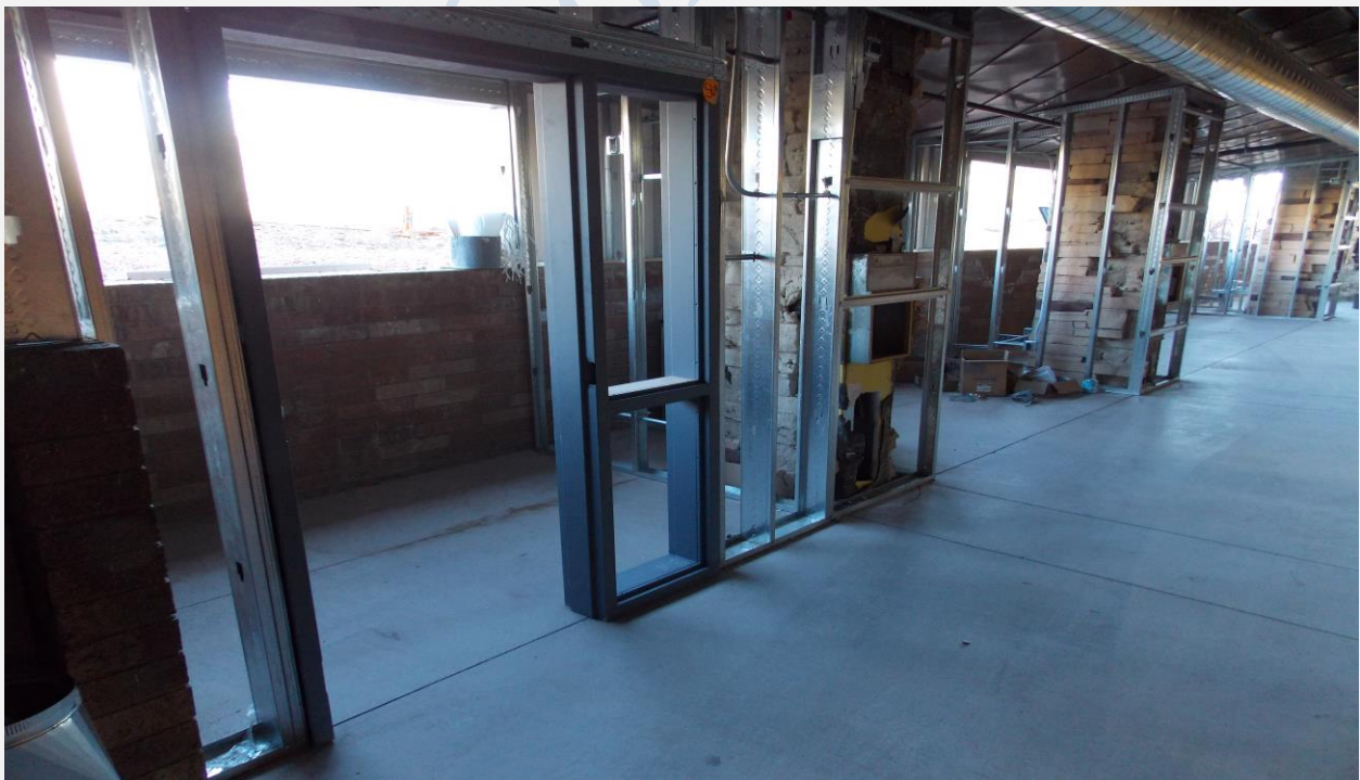
Framing of Office and Student Break Out Rooms - First Floor
